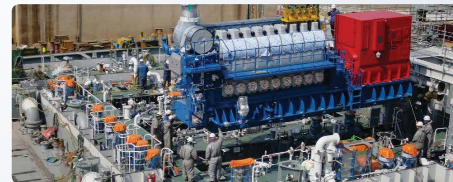
One of six HIMSSEN 9H32 engines being installed
